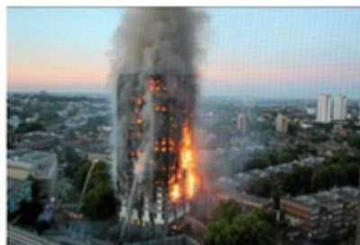
The 2017 Grenfell Towers fire in London has sparked a costly audit of all Queensland buildings of three floors or more.
