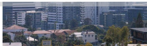
PHOTO: It is not known how many non-government buildings in Queensland have the unsafe cladding (ABC News: Isobel Roe)
